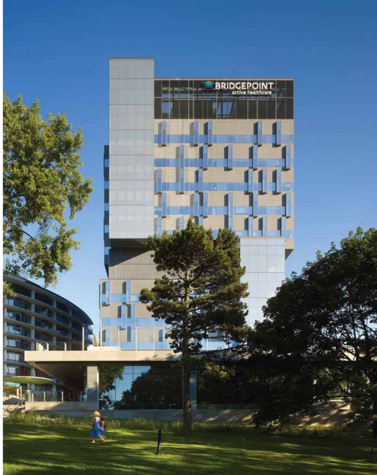
View of North Facade from Riverdale Park. Photo: Tom Arban
