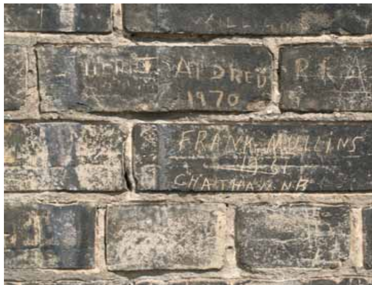
Original buff bricks, complete with graffiti were painstakingly restored. Photo: Stephen Phillips
